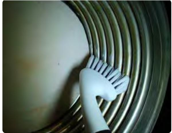
9. Wipe any residue off coils with a clean rag.
