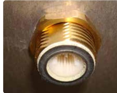
6. Combi Boiler: Domestic water inlet connection showing filter screen to protect paddle flow switch from sand and other debris.
