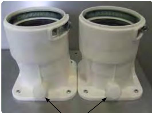
Vent and Air adapters to be installed with test ports facing to front of boiler. Must be locked closed.
