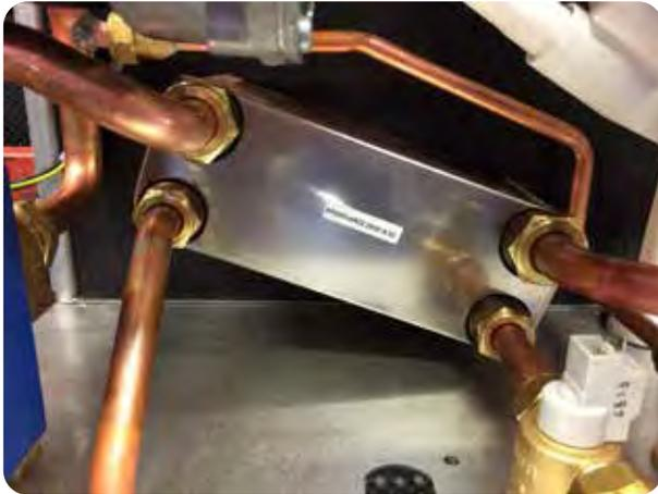
5. The treatment time must be chosen according to the amount of scale deposits present in the exchanger and however such time must always be less than the maximum treatment time specified by the manufacturer on the product data sheet.
