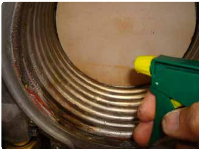
8. Lightly spray clean water on all of the boiler coils and clean any residue off with (plastic only) brush. (Be careful not to damage back refractory wall).
