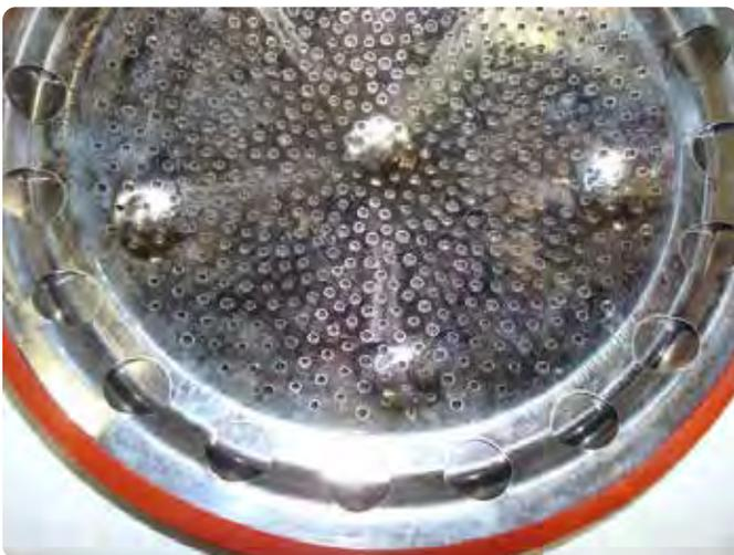
6. **Inspect the interior of the burner. Brush and vacuum the interior if needed to remove lint or sediment. Alternative cleaning methods:**
