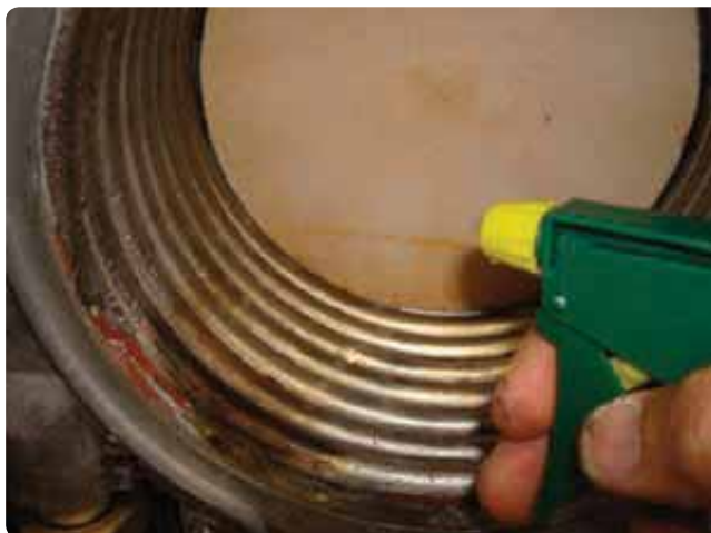
Figure 145 Cleaning the heat exchanger
