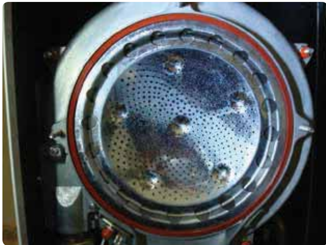
Figure 141 Inspection and removal of burner and gasket
