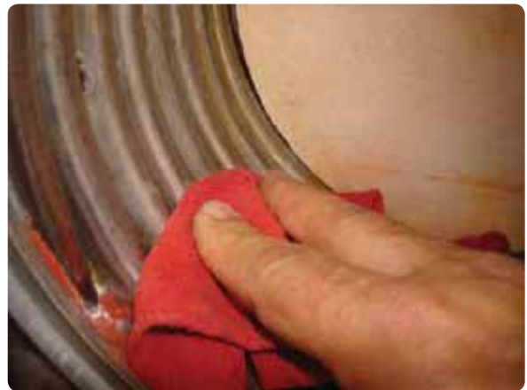
Figure 147 Cleaning the heat exchanger
