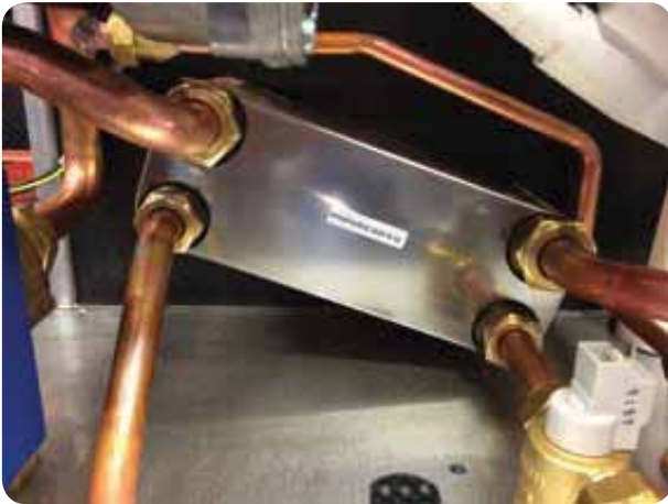
Figure 155 Removal of flat plate heat exchanger by loosening the four fittings. Combi-155
