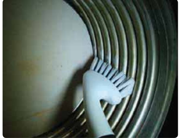
Figure 146 Cleaning the heat exchanger
