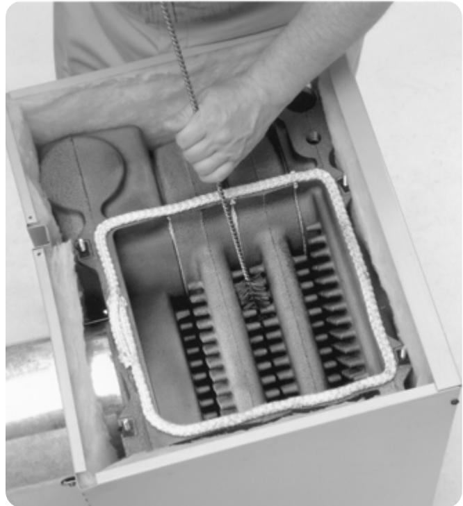
**▲WARNING** Wear a NIOSH -certified dust respirator (N95) while cleaning the boiler, per WARNING on page 25. Failure to comply could result in severe personal injury.
