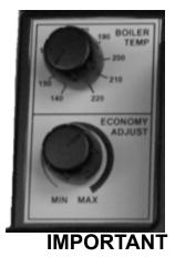
In accordance with Section 325 (f) (3) of the Energy Policy and Conservation Act, this boiler is equipped with a feature that saves energy by reducing the boiler water temperature as the heating load decreases. This feature is equipped with an override which is provided primarily to permit the use of an external energy management system that serves the same function.
